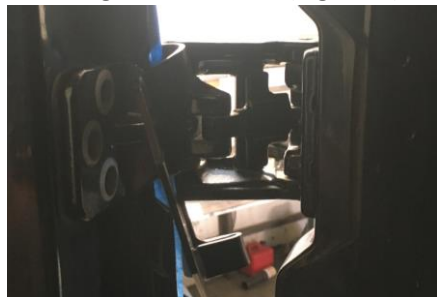
Figure 4: Hinge Placed Back into Position
