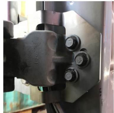
Figure 6: Inside View of Installed Lower Hinge Bracket
